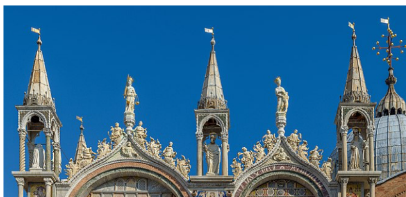
Detail of the south facade of St Mark's Basilica
